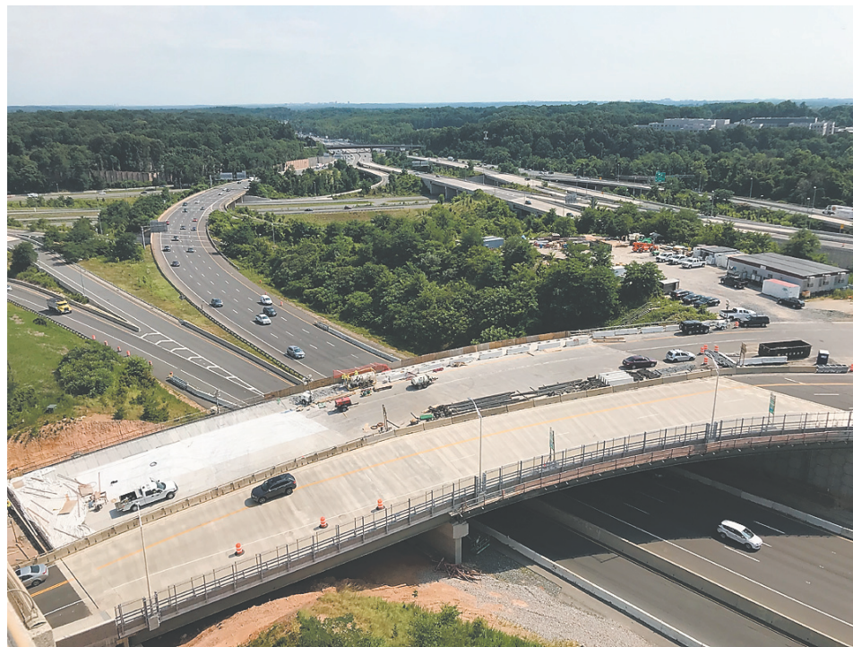
PHOTO COURTESY OF VDOT
